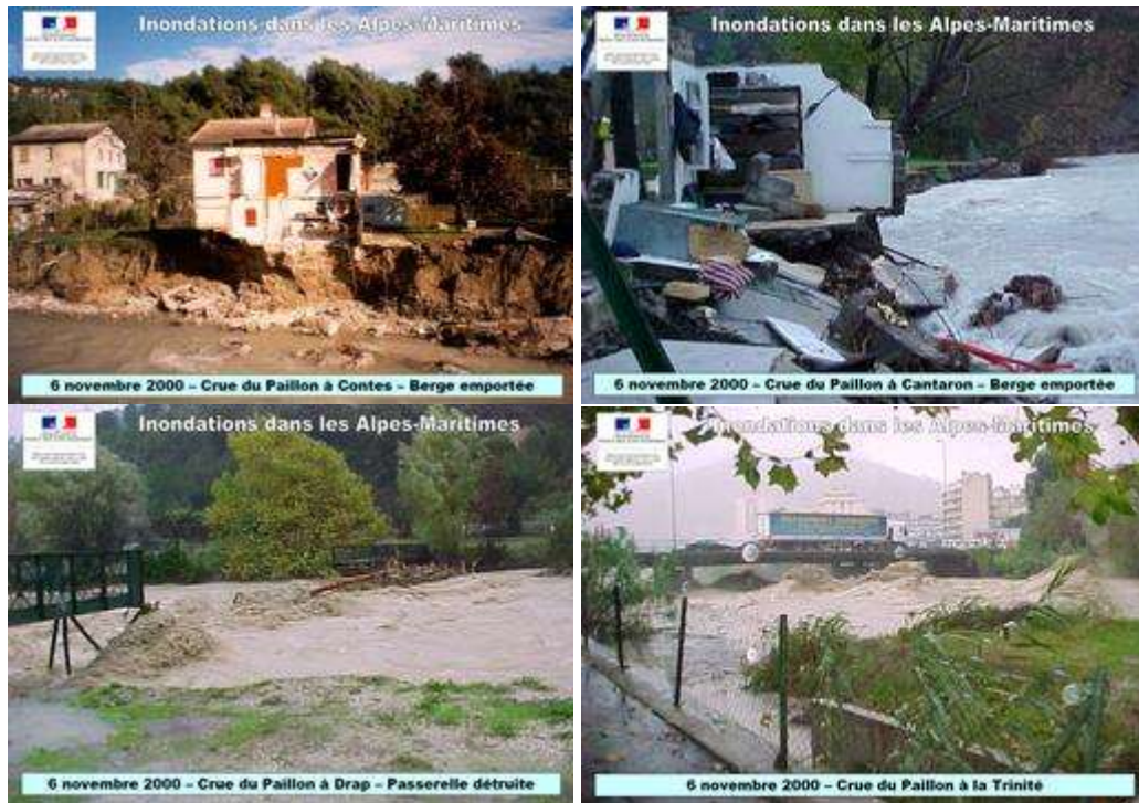
Figure 31 Damages of flood of November 6 th ,2000 in the Paillons upper valley ( www.cypres.org ).
